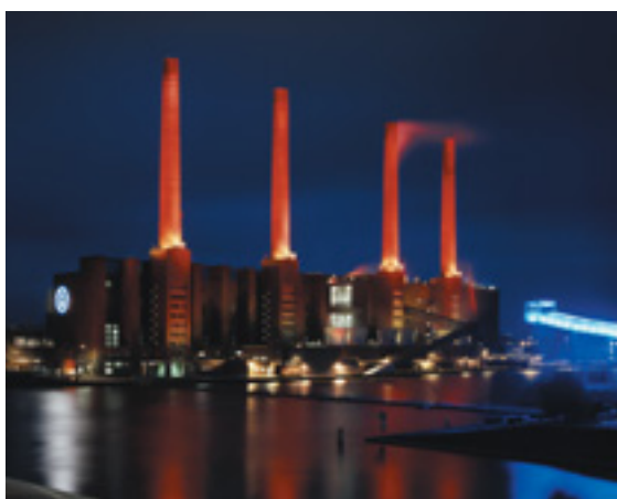
Photo: A & O Lighting
