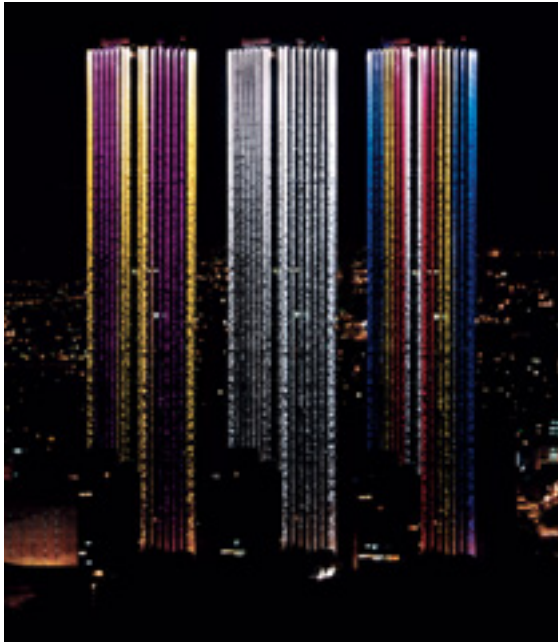
A spectacle in light with XBO® 3 and 4 kW. Roof-mounted spotlights create colourful effects on the 200 metre high façade of the Bogotá Tower in Columbia.
